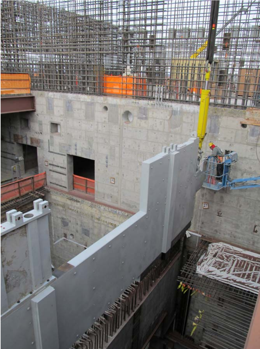
(Photo 2 of 2) The 102-ton shield door measures 52 feet wide and 15 feet tall.
