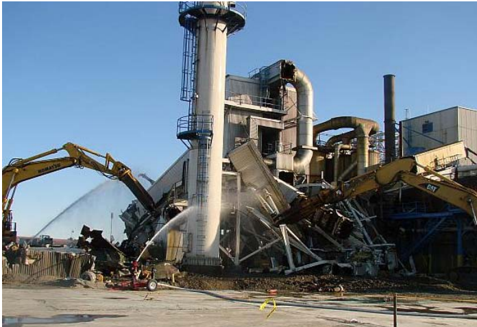
Workers demolished the 384 Building in 2008.
