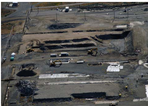
Cleanup of the 618-1 Burial Ground was part of a TPA milestone.
