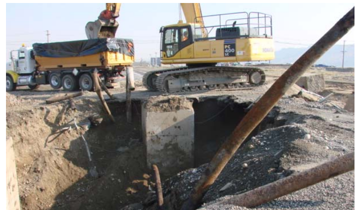
More than 8,000 feet of pipe was removed from 300-15. Facilities associated with the process sewer line dumped beryllium liquid waste down drains, creating challenges for the cleanup team.
