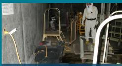
Workers are removing radiological and chemical hazards from inside the REDOX canyon to prepare the facility for eventual demolition.
