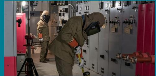
*Electrical isolation ensures worker safety as the PUREX canyon is prepared for demolition.*
