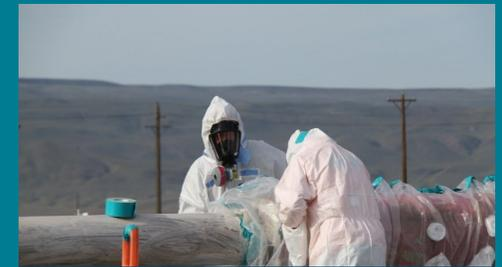
*Workers are removing hazards such as asbestos from about 1,700 feet of old steam lines at the PUREX facility.*
