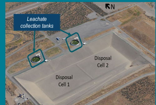
Workers will monitor, collect and treat leachate in two large tanks.
