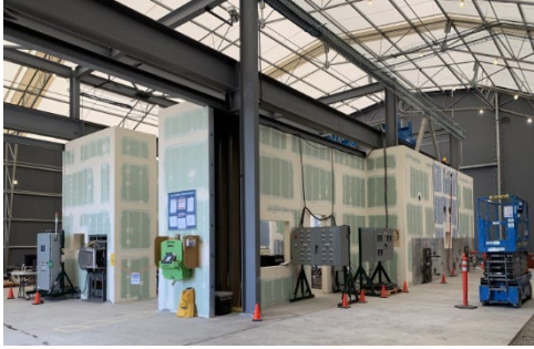
Workers constructed a mock-up to replicate features inside the 324 Building.
