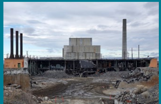
Demolition of 165 K West powerhouse, January 2022.
