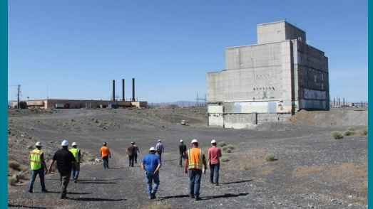
Below: K East Reactor building in 2020 before cocooning.
