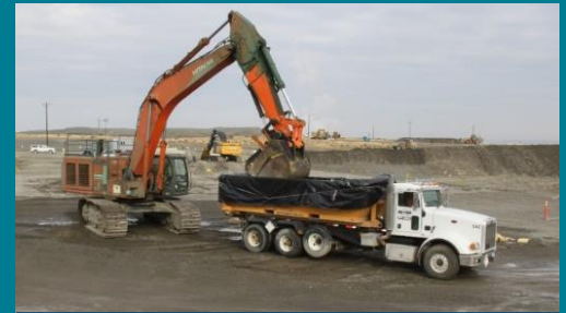
Containers are filled with waste to be disposed of at the Environmental Restoration Disposal Facility.
