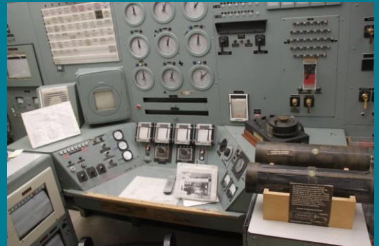
The control room inside B Reactor.
